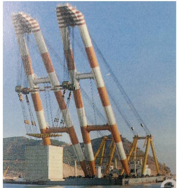
Lowering the caisson built on land to the sea with a 2,000-ton-class maritime crane
