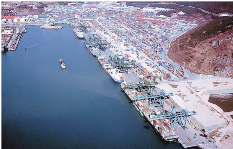
Expanded Terminal as of November 1997: Ssangyong E&C executed the additional construction project to expand the pier to allow simultaneous birthing of four 50,000 tonnage ships (From November 1997 to May 1995)
